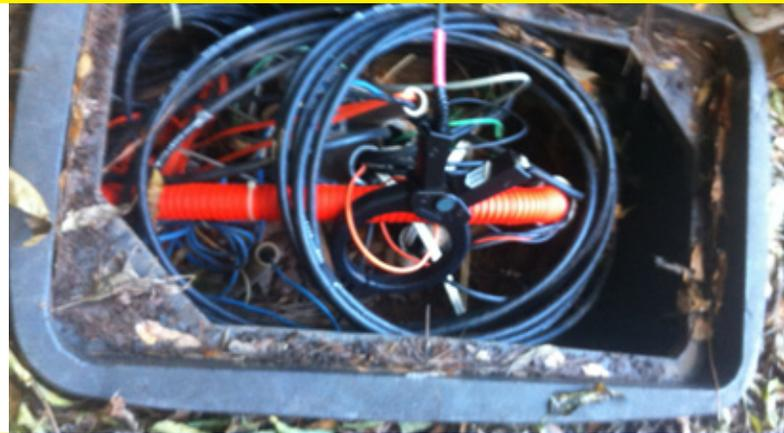
**2ND CHOICE – Close Induction Technique:** If direct connection is not possible or does not give you the results you need, the use of an induction clamp (coupler) is the second most effective method of applying a locate signal onto the target line. This method limits the choices of broadcast frequency and power outputs when compared to direct connection. The close inductive coupler, commonly
