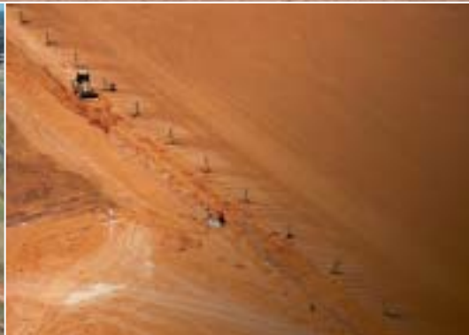
Major earthworks in progress to create one of the holding basins
