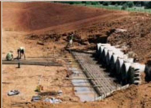
Constructing seven 1,050 mm diameter culverts to an instream basin
