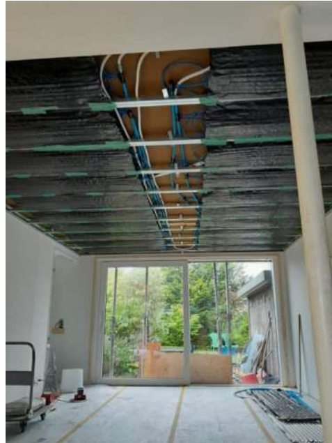
Kühldeckenpaneele in Abhangdecke
